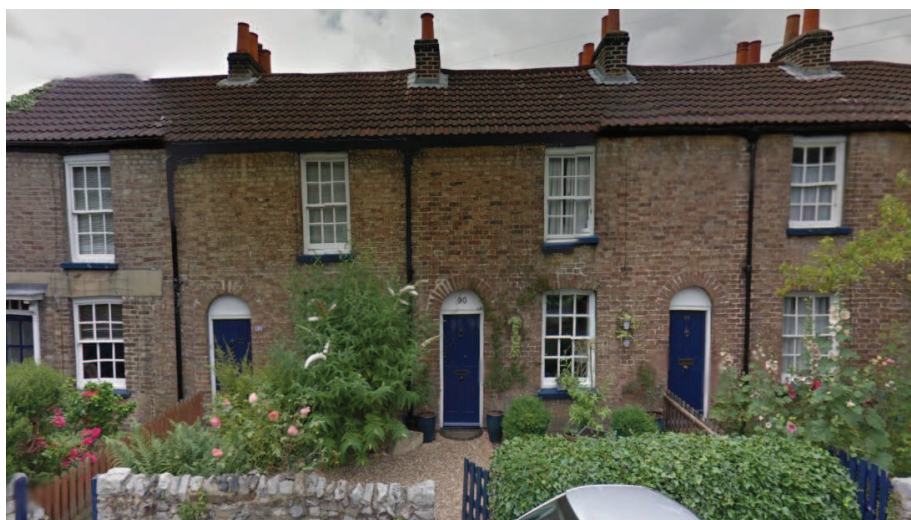
84-94 Phipps Bridge Road
